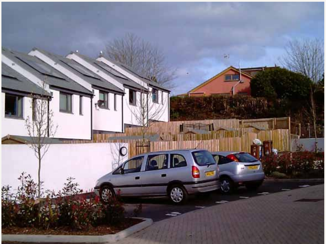
As a result of its tree policy, Tor Homes's new development include good tree planting provisions. © Tor Homes
